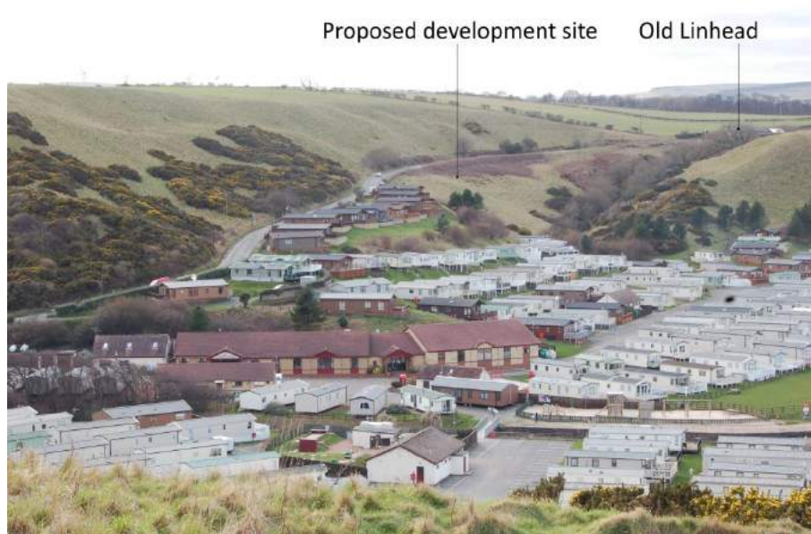
Figure 6.7 The existing lodges in the upper part of the site are less prominent than those in the lower levels, due to different colouring.
